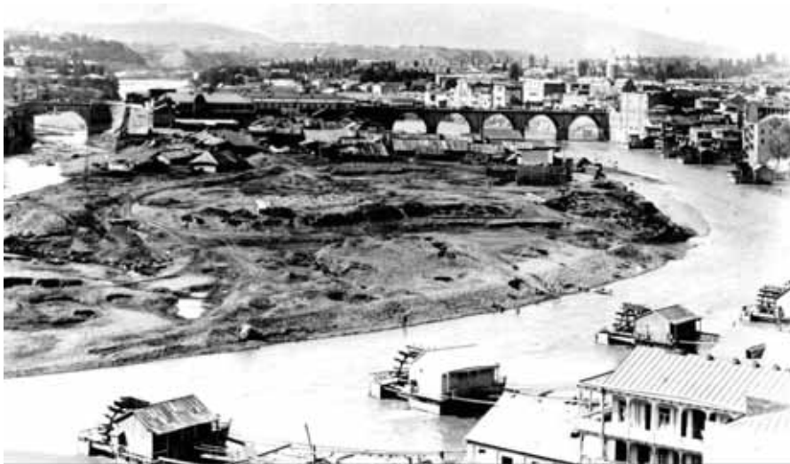
The historical Madatov Island, today the site of the Justice Palace. In the background stands the Dry Bridge, then called Mikheil's Bridge.
