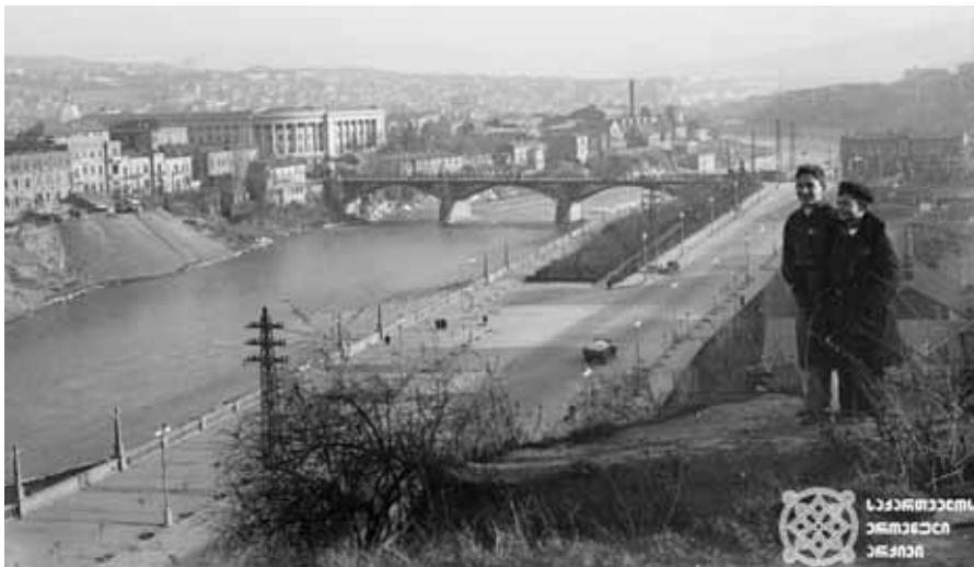
A view of the then newly constructed right embankment highway from Vere Park. The left embankment highway has not been constructed yet.
