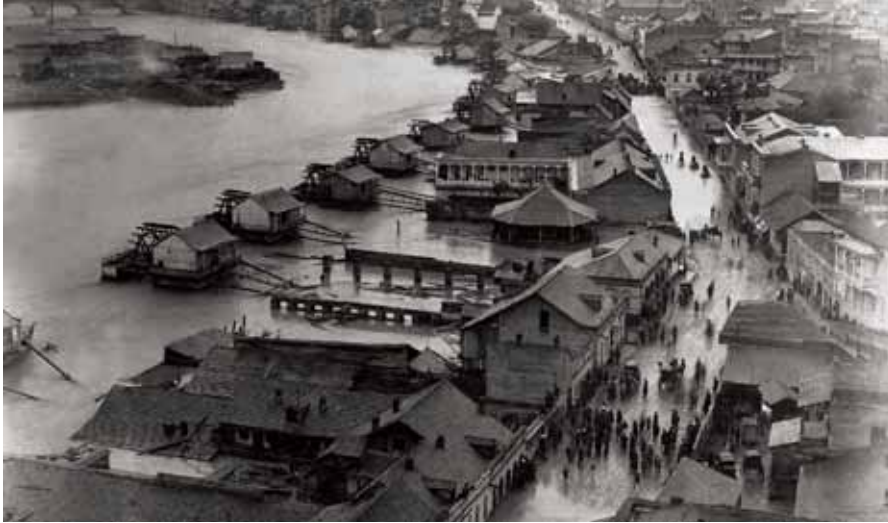
Floating waterwheels on the Mtkvari historically provided power for mills and other kinds of workshops until they were demolished for the construction of the embankment highways.
